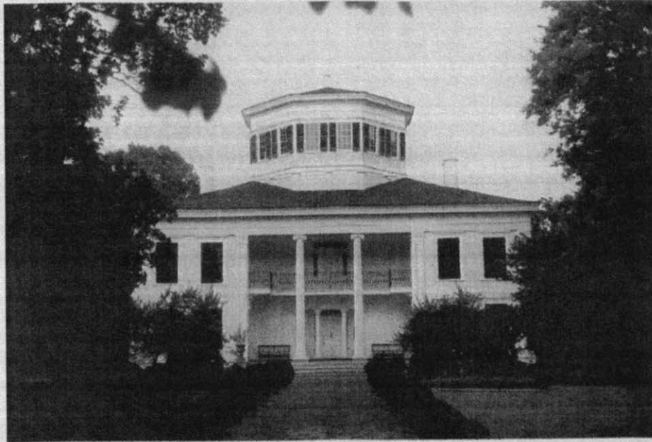
Figure 3. Waverly Mansion, West Point, Mississippi. Completed in 1852.
